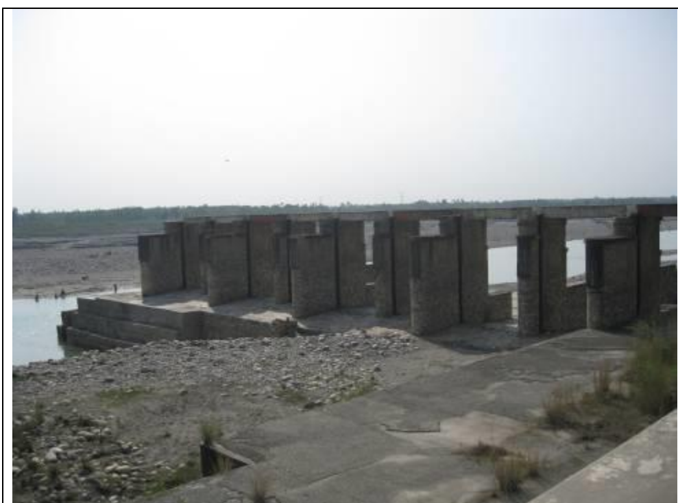
Photo 4: Tajewala Barrage supplying to Western Yamuna Canal
