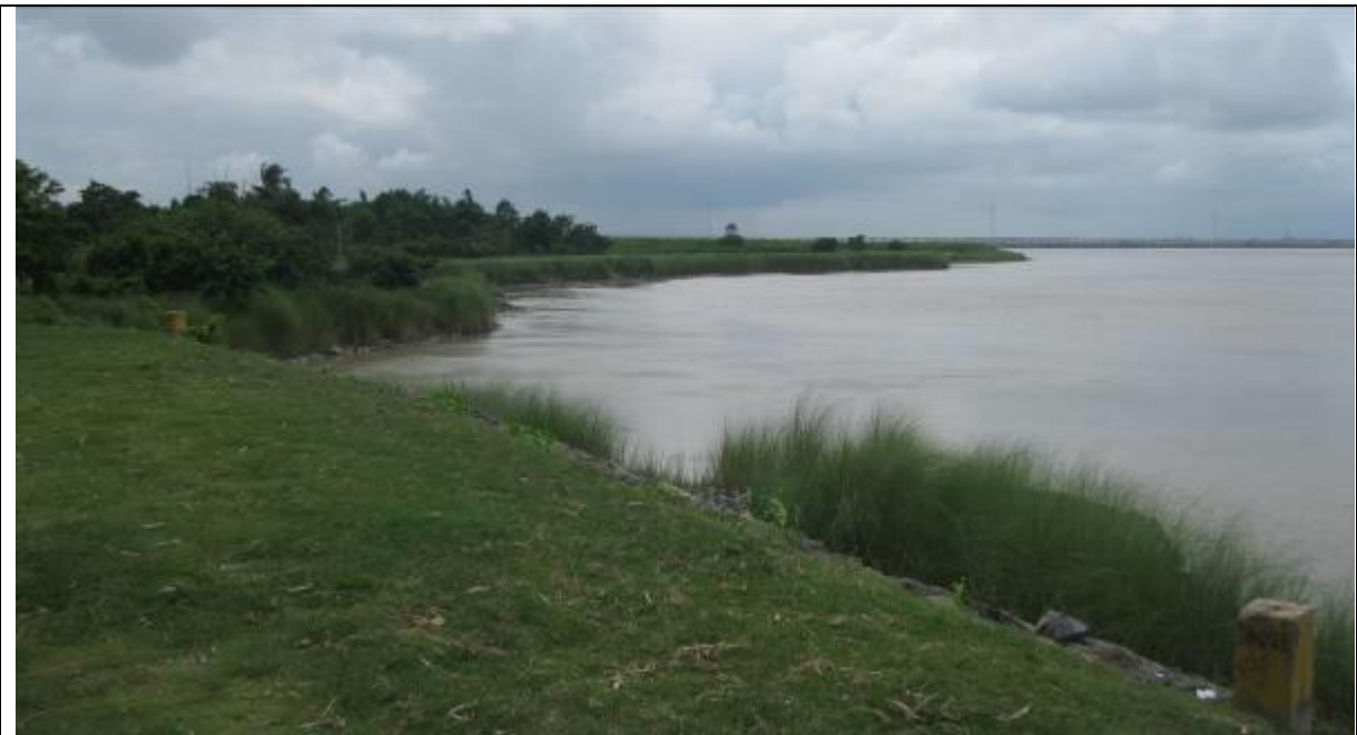
Photo 1: Erosion on Left Bank upstream of Farakka. A village used to exist here.
