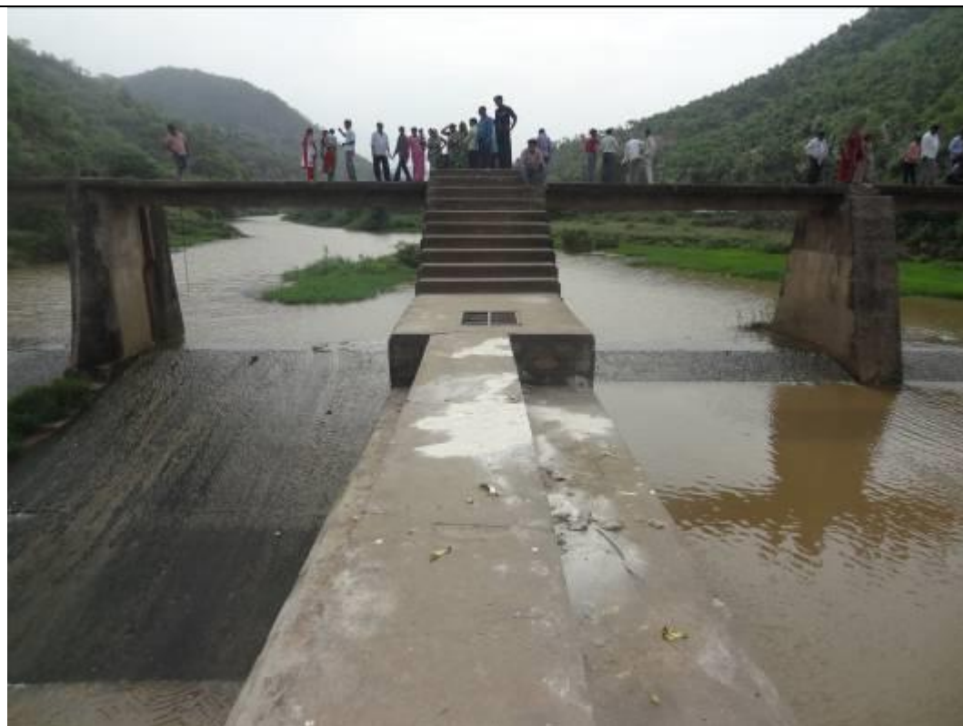
Photo 5: Structure on Ruparel River
